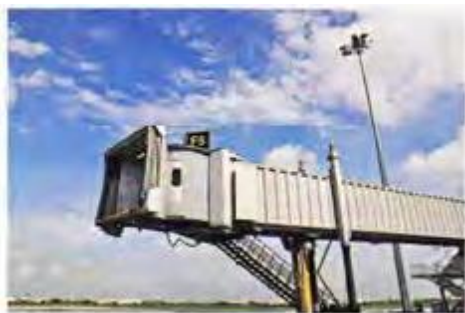
4 Loading Bridge(Jet Bridge)
